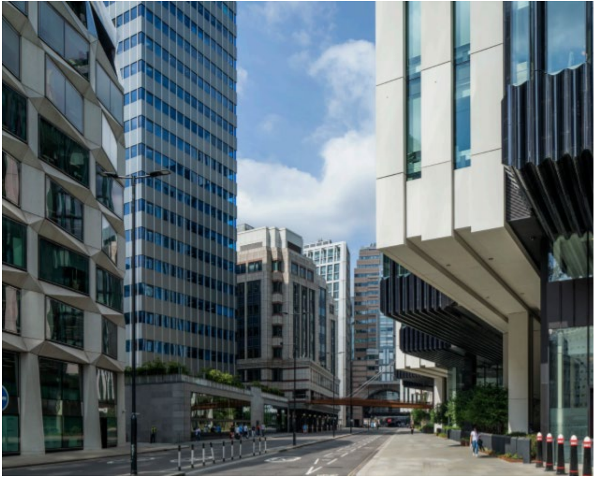
City Tower and City Place House looking west along London Wall
