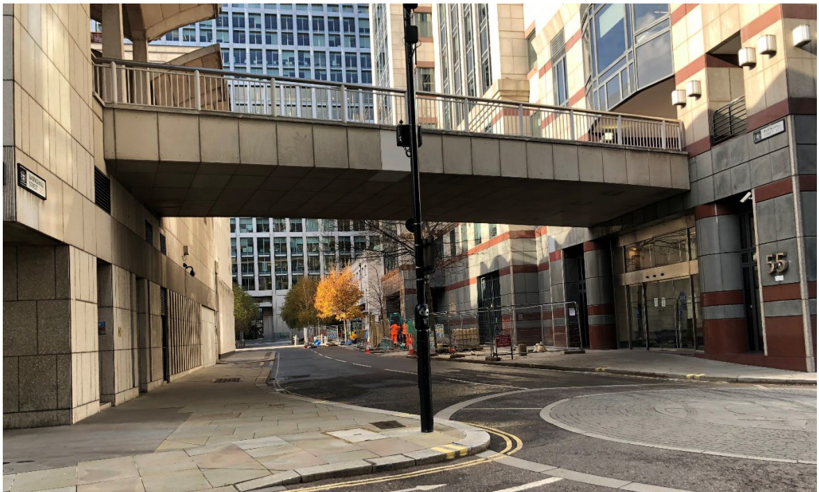
Walkway Bridge between 65/65a Basinghall Street and City Place House (looking west along Basinghall Street)
