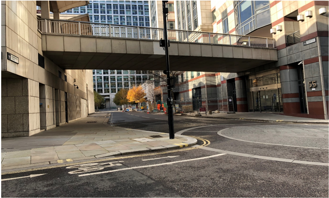
Walkway Bridge between 65/65a Basinghall Street and City Place House (looking west along Basinghall Street)
